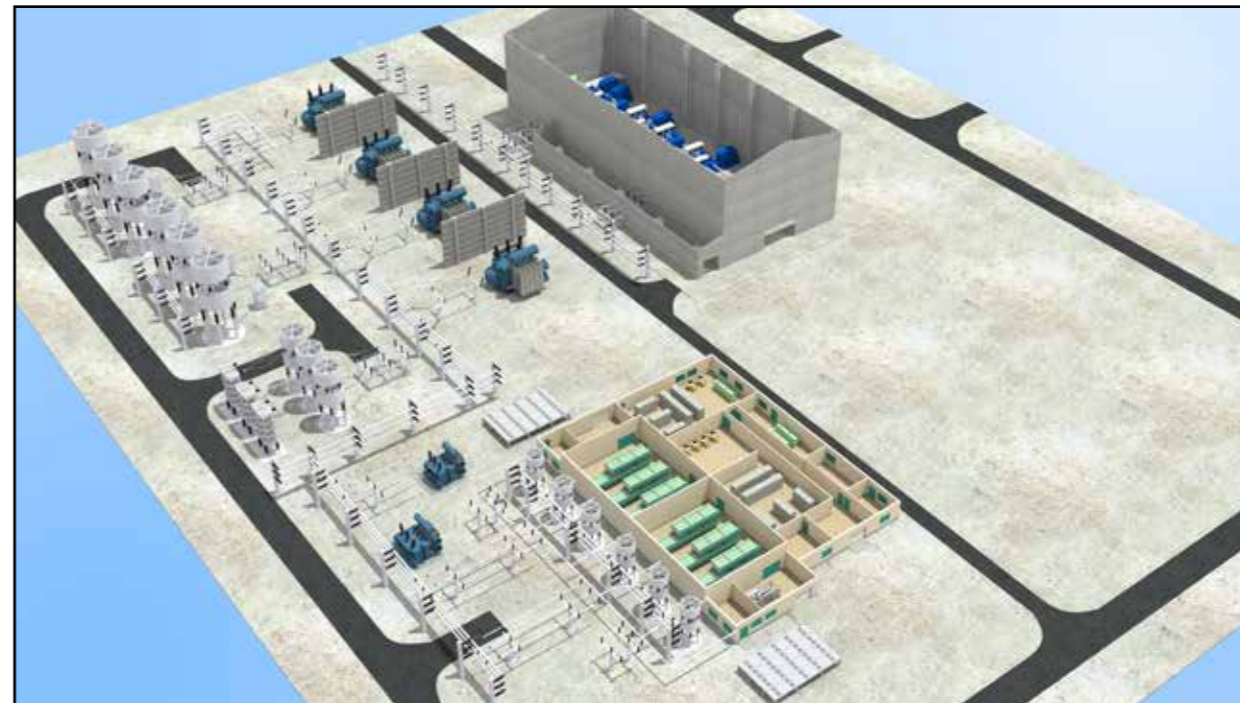
Figure 3: 3D model of an upcoming STATCOM station in India (Courtesy: Montnets Rongxin Technology Group Co., Ltd)
