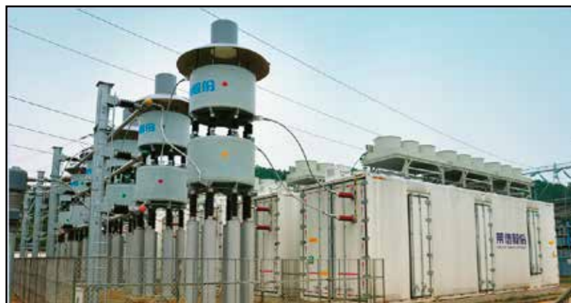
Figure 1: ± 200MVAR, 500kV, outdoor containerised STATCOM system (Courtesy: Montnets Rongxin Technology Group Co., Ltd)
